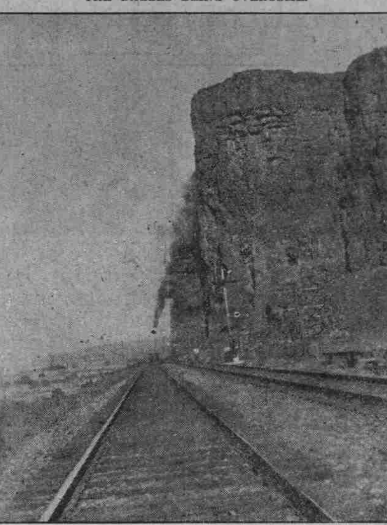
CAPE HORN BEING BLASTED TO MAKE WAY FOR ROAD. The view shows Cape Horn, which is being partly blasted away to make room for the highway. A tunnel through this mass of stone was found unsafe on account of the formation, and it was found necessary to blast the road along the side of the rock above the railroad. Great care has had to be observed on account of the proximity of the railroad. This great rock is located on the south bank of the Columbia river between The Dalles and the Deschutes river and should not be confused with the Cape Horn on the north side of the river opposite Crown Point.
